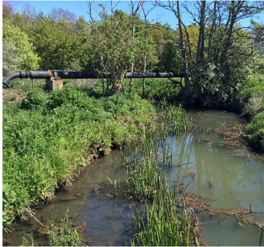
River Alde upstream of the proposed bypass
